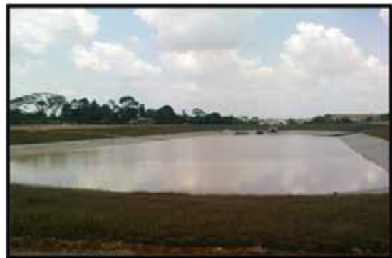
Kolam Takungan Hospital Permai
