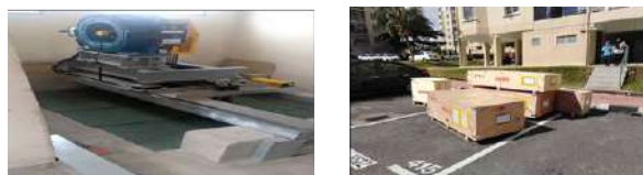
Gambar 4.8 : Kerja Projek Lift Plot C Larkin Idaman, MB Johor Bahru.
